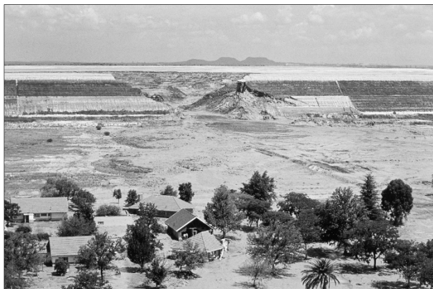
Fig. 6 The devastation of the mudflow following the Merriespruit tailings dam failure, South Africa (February 1994).
