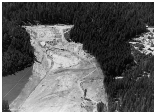
Fig. 5 The failed dams and the devastation of the Stava valley (July 1985).
