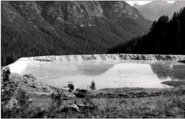
Fig. 2 View of the Stava lower basin in 1969.
