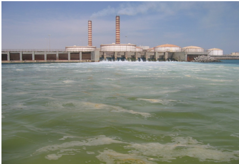
Fig. 2 Az-Zour desalination plant and outfall structure.
