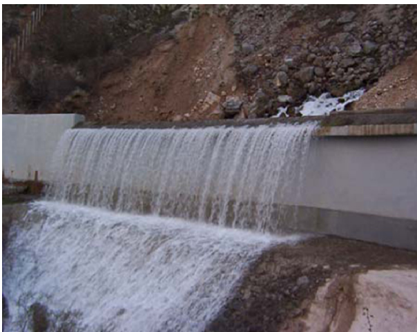
Fig. 3 Photo of dam in catchment facility.
