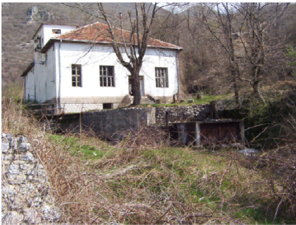
Fig. 8 Photo of hydropower building.
